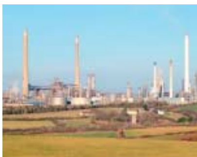
Figure 6.14 Texaco Oil Refinery, Pembroke, Wales
